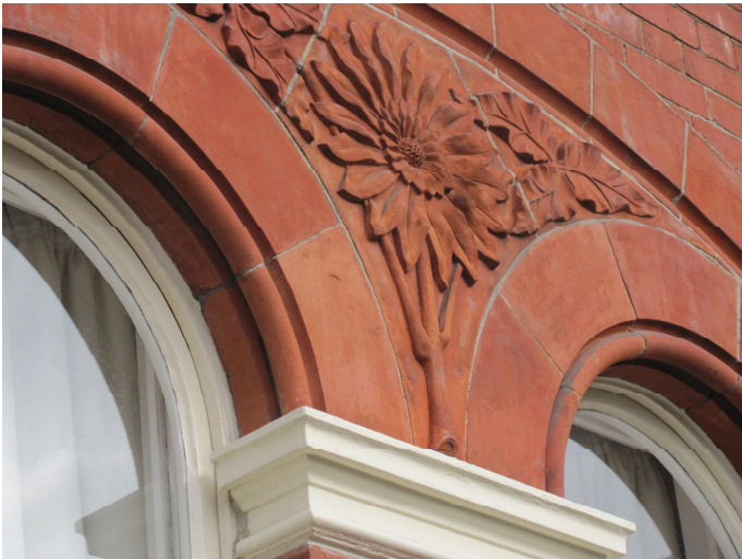
Completed specialist brickwork repairs, façade cleaning and redecoration.
